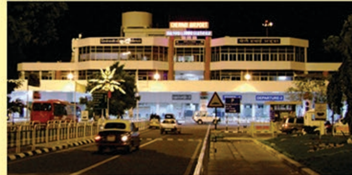
National Terminal Complex, Madras Roof insulated with DUGAR INSULSET ROOF INSULATION
